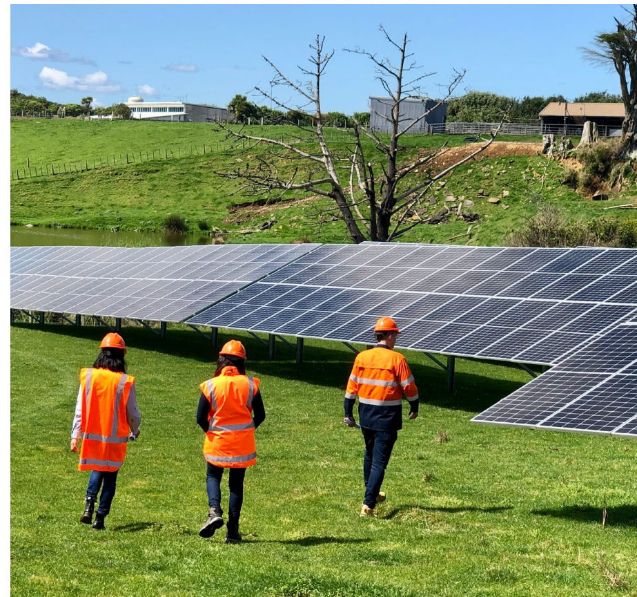
Above: Todd's Kapuni Solar Plant in South Taranaki
