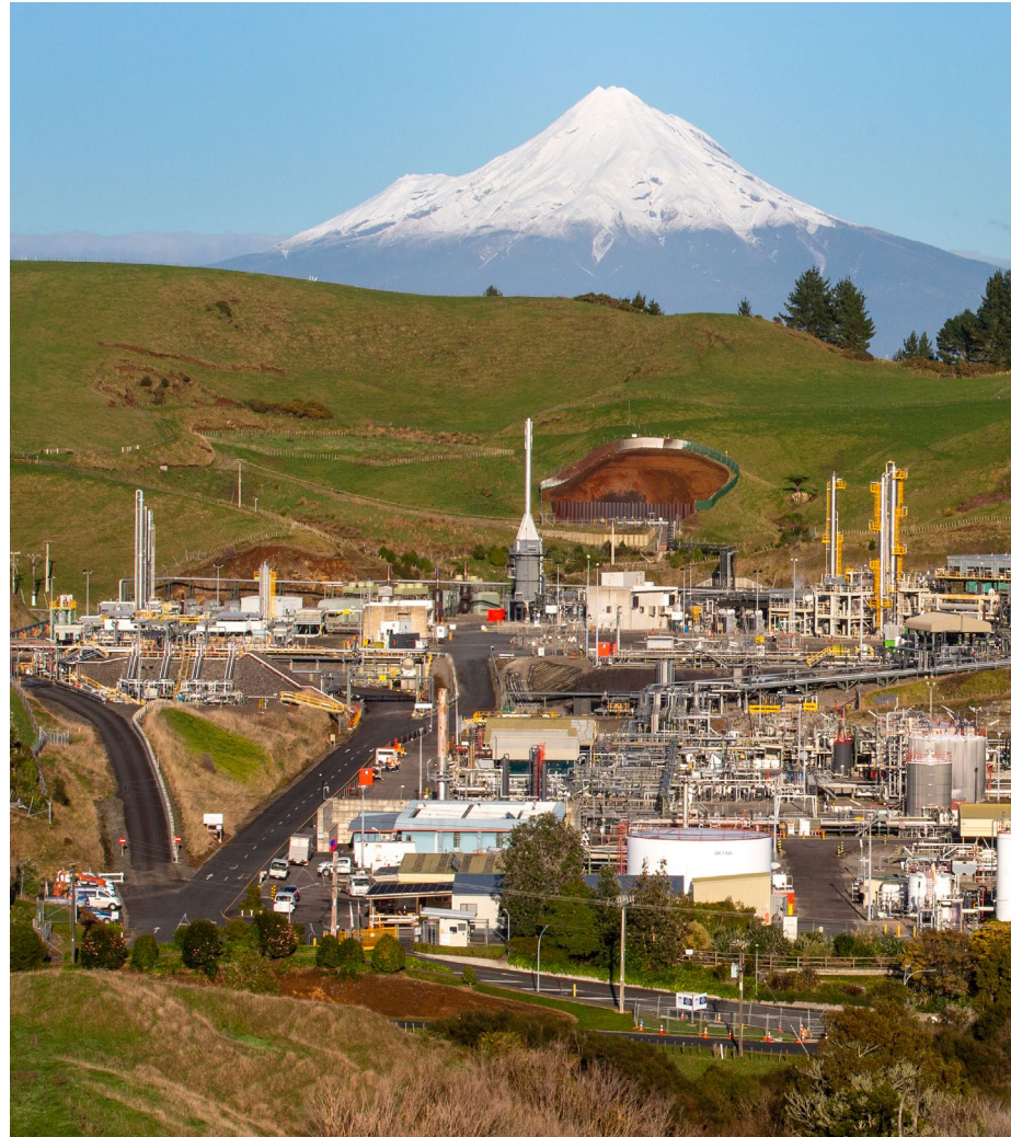
Right: Todd's McKee Mangahewa Operating Facilities in North Taranaki
